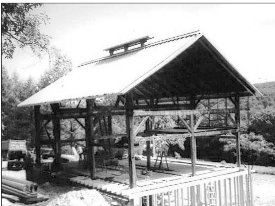
...during the renovation...
